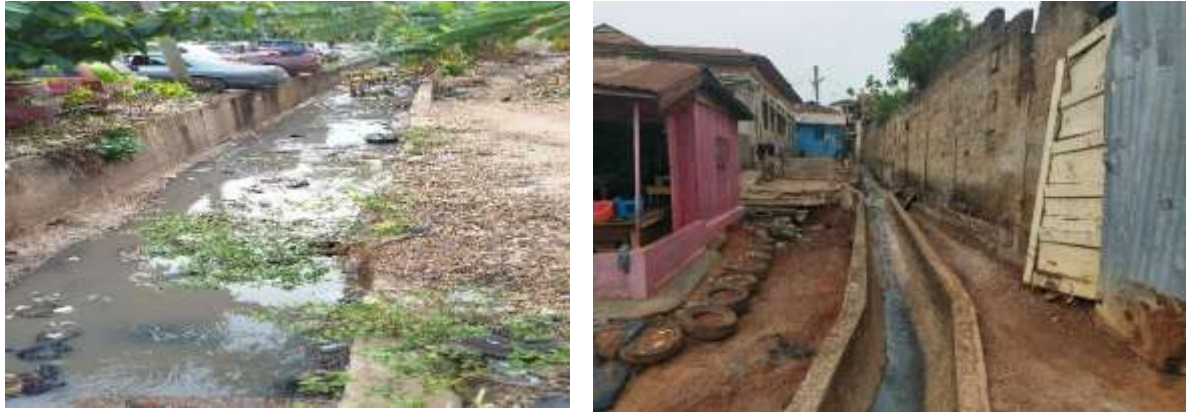
Fig. 6 Some drains in Kumasi (photographed by a Research Assistant, 2024)
